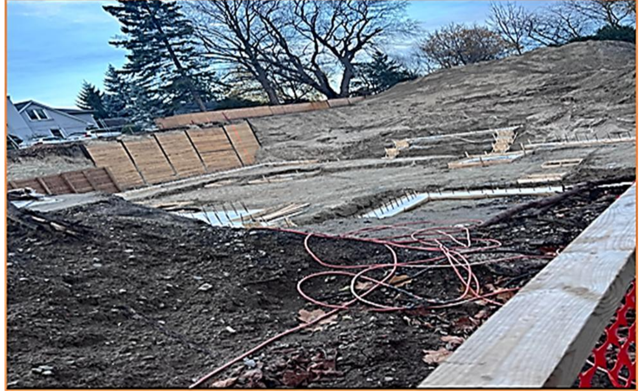
Image of site currently under construction in 2025
